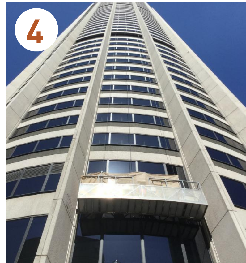
PRECAST CONCRETE VERTICAL HOTEL BLADES
