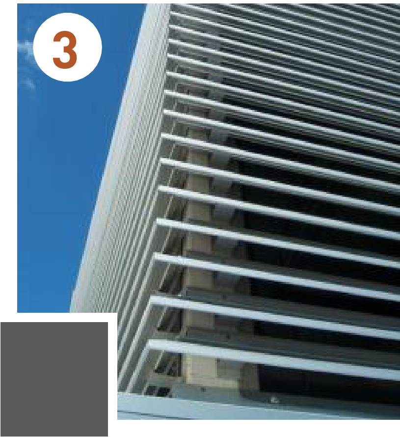
LOUVRED FACADE CHARCOAL PLANT & LIFT CORE
